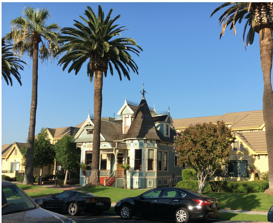
Figure 3. Note the one-story configuration of the new construction at the side elevations of the historic building and the generous setbacks of the new construction.
