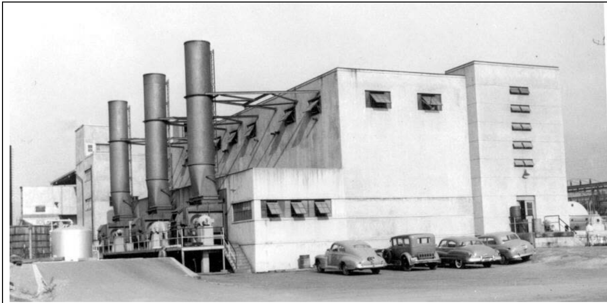
Figure 4: Grayson Steam-Power Plant Building, view northwest of south endwall, circa 1950s. Source: https://commons.wikimedia.org/wiki/File:Grayson_Power_Plant.jpg , not for publication.
