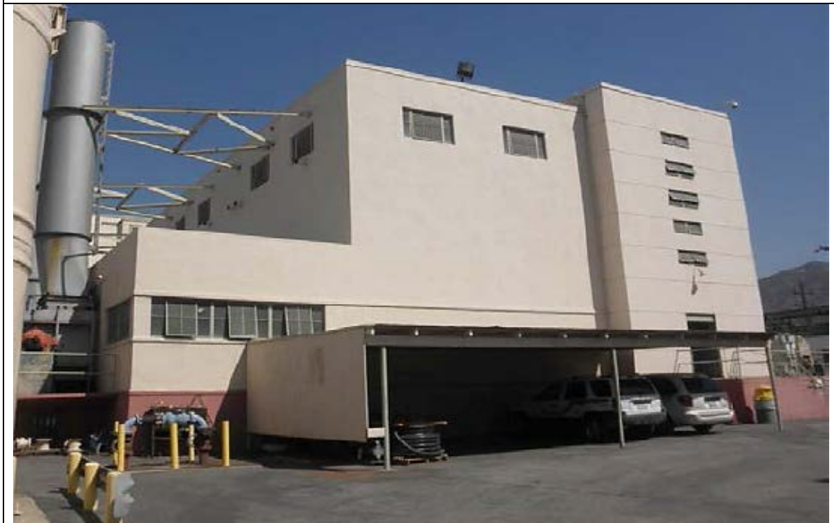
Figure 5: Excerpt from Initial Study, Architectural Resource Evaluation Of The Grayson Power Plant For City of Glendale, California, undated photograph estimated 2016, (Figure 26 Grayson Boiler Building page 6.10, same view as Figure 4 above). Note all visible awning-type, steel sash windows, exterior materials, the building configuration and Stripped Classicist design remain recognizable. Carport at lower center is an addition (year unknown). Note the stucco scoring bands at the right-hand boiler building tower and the dimensioned continuous sill and header on the left-hand bank of ribbon windows that enunciate the endwalls, providing visual interest and relief. Other than the carport, no alterations are visible.
