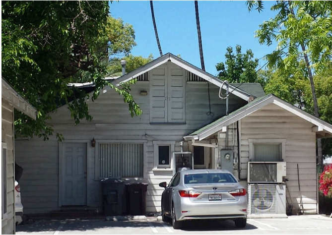
Figure 2. View east of the rear of the house at 128 S. Kenwood, showing hay loft, five-panel doors at the apex of the main gable. The hay loft doors are flanked by decorative attic vents on either side.
