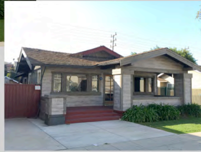
Unpermitted alterations at right Nov. 11, 2017
