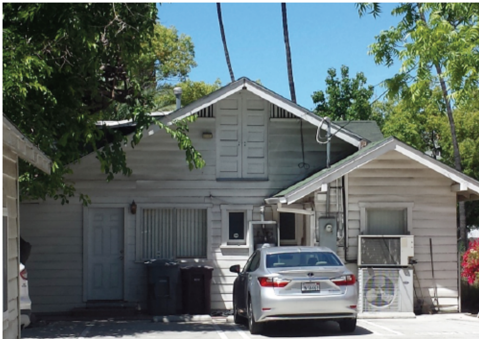
Figure 1. View east of the rear of the house at 128 S. Kenwood, showing hay loft, five-panel doors at the apex of the main gable.
