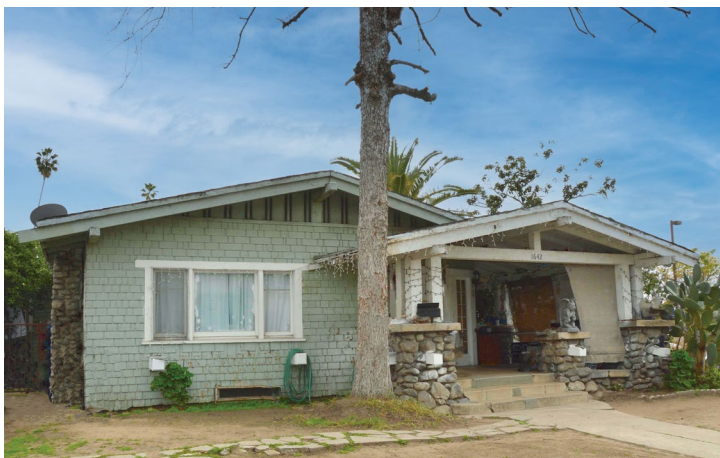
1642 S. Central, a Mills Act-eligible property slated for demolition
