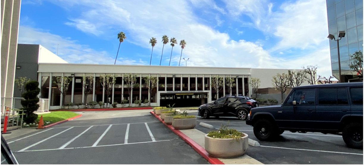
Figure 1: Parking Garage at 620 North Brand Boulevard, view east. Note the simple base, filleted shaft separated by screens and the bracketed, wide upper frieze. The stepped out, framed entry portal on the right-hand side further echoes the Corporate Modern design style of the main building it was constructed to serve. Photograph January 2022.
