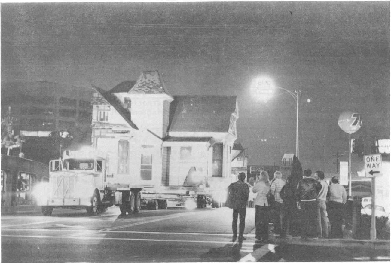
The two sections of the Doctors' House approach the junction of Central and Glenoaks, drawn by the powerful trucks of Ability Movers and watched by members of the Society, telephone company employees and curious nightbirds. (Photo by Sid Gordon)
