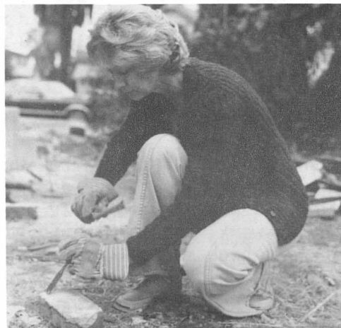
Restoration work began from the ground up.
