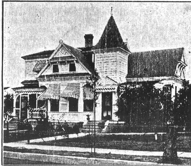
Residence of Dr. L. H. Hurtt T on Third avenue, Glendale.
