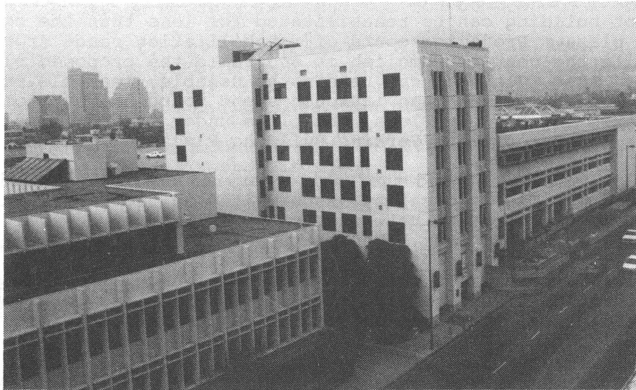
The Public Service Building (center) is flanked by the Municipal Services Building (left) and the new C.E. Perkins Building (right; under construction). The buildings, built approximately 30 years apart, are aesthetically compatible and demonstrate a significant evolution of building styles.
