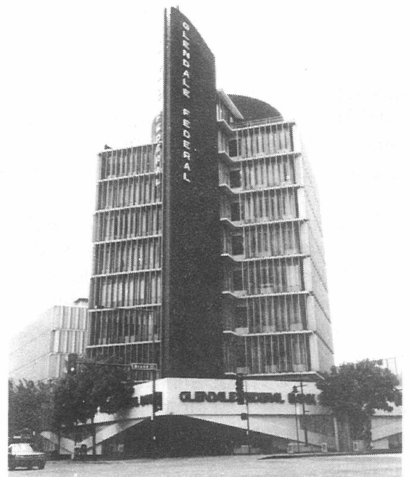
The Glendale Federal Building 401 N. Brand Blvd. in 1998, before the title letters were removed from the fire tower.
