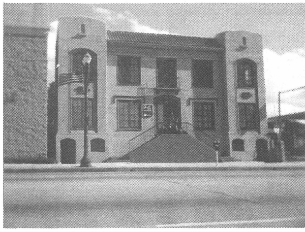
This is the apartment complex that will be demolished.
