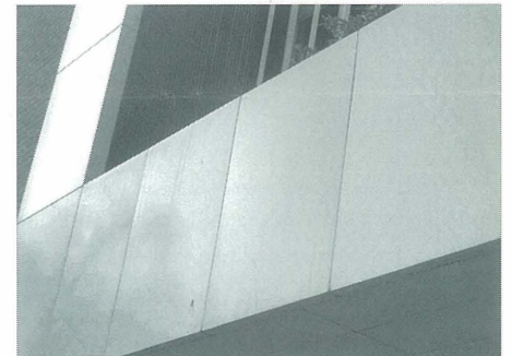
Detail of the Fidelity Federal front facade
