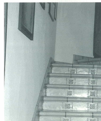
Restoration Completed: Original designs and stamped stair risers on 1930s stairway and wrought iron railing with the original finish restored
