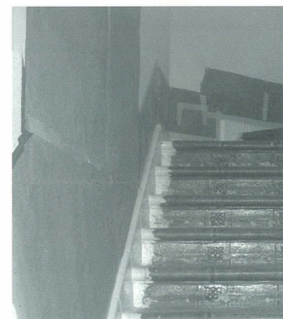
During restoration: Magnesite under the carpet was ravaged by nail holes
