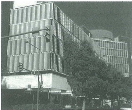
Annex before removal of louvers
