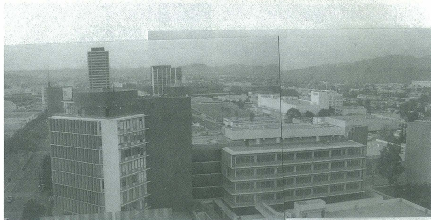
A view of GlenFed Annex from the building across the street before the removal of its louvers. A photo on page 4 shows the Annex without louvers.
