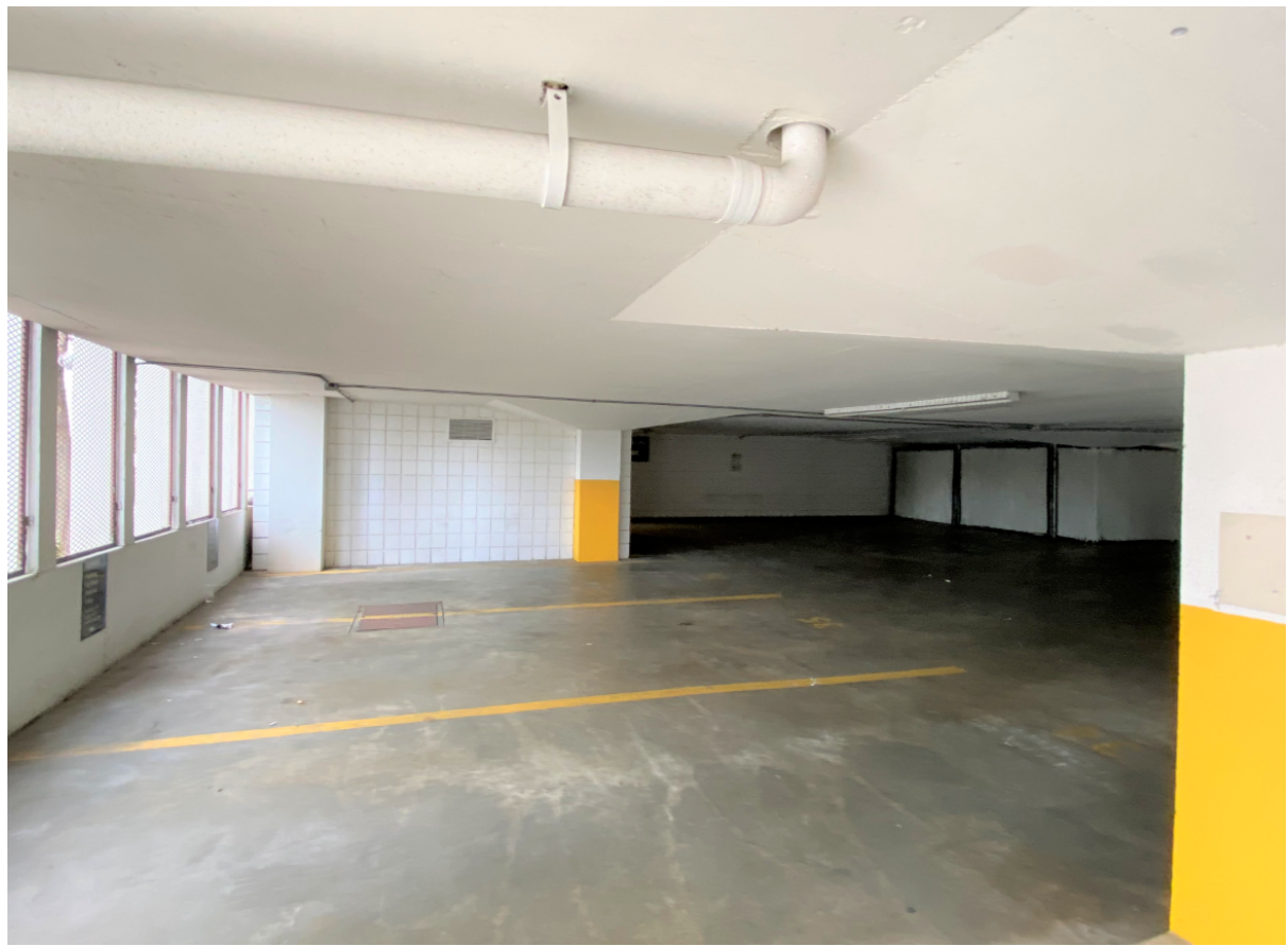
Figure 2: Parking Garage interior view north. Note the fitted screens in the exterior openings (left) archaic stack bond endwalls (center and right), and square, full height support columns at center and right with yellow bases. Photograph January 2022.
